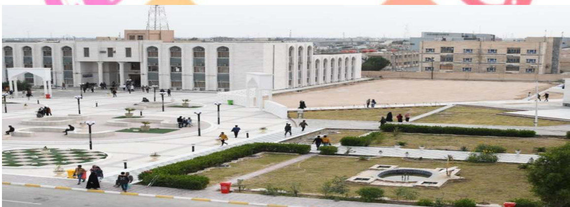
Samawa site buildings
