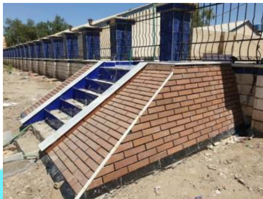
16. Making iron awnings in the yards.
