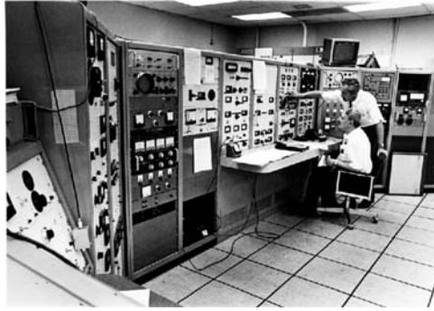
Fig. 16.1. A “knob-based” central control console used to control the High Voltage Engineering Corporation model FN tandem accelerator and associated components at the Triangle Universities Nuclear Laboratory, Duke University, Durham, NC. The photo is circa 1970 and courtesy of Chris Westerfeldt, TUNL, Duke University
